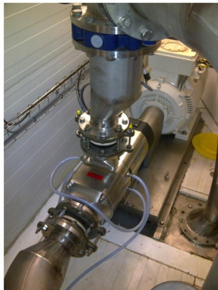
HYGHSPIN 125 pump with base plate assembled on a fruit juice tanker
